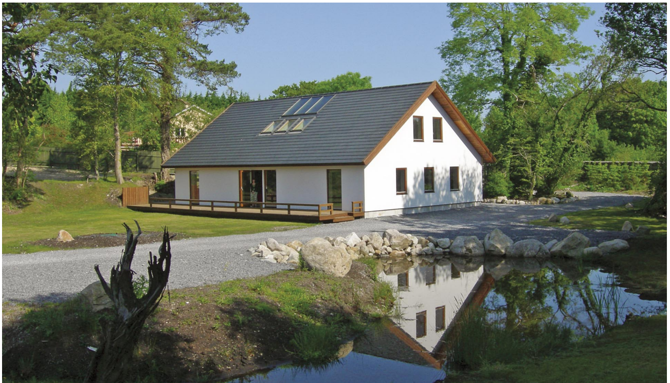
Passive house built in Galway, Ireland, by Scandinavian Homes Ltd. 250m 2 floor area and six bedrooms. A minimal heat requirement of <math><3\text{watt per m}^2\text{ floor area}</math> in the mild Irish winters. Timber frame construction. Evaluated by Passiv Haus Institute programme PHPP
