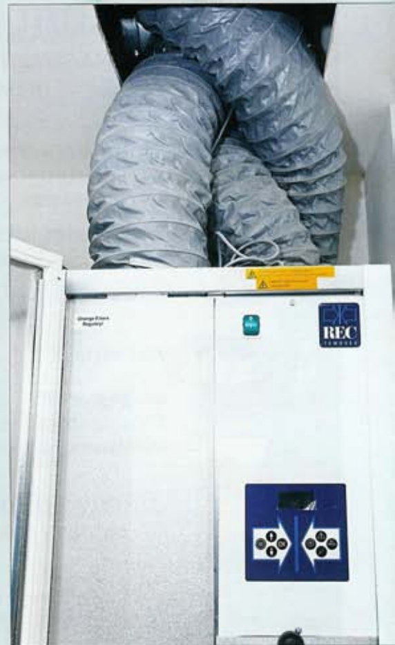
(clockwise from top left) The house's simple cube shape is designed to reduce the surface area and minimise heat loss; an automatic floor sander smooths the solid timber floors; a heat recovery unit ventilates the house; the house's timber windows are triple-glazed and argon-filled with a low-e coating
