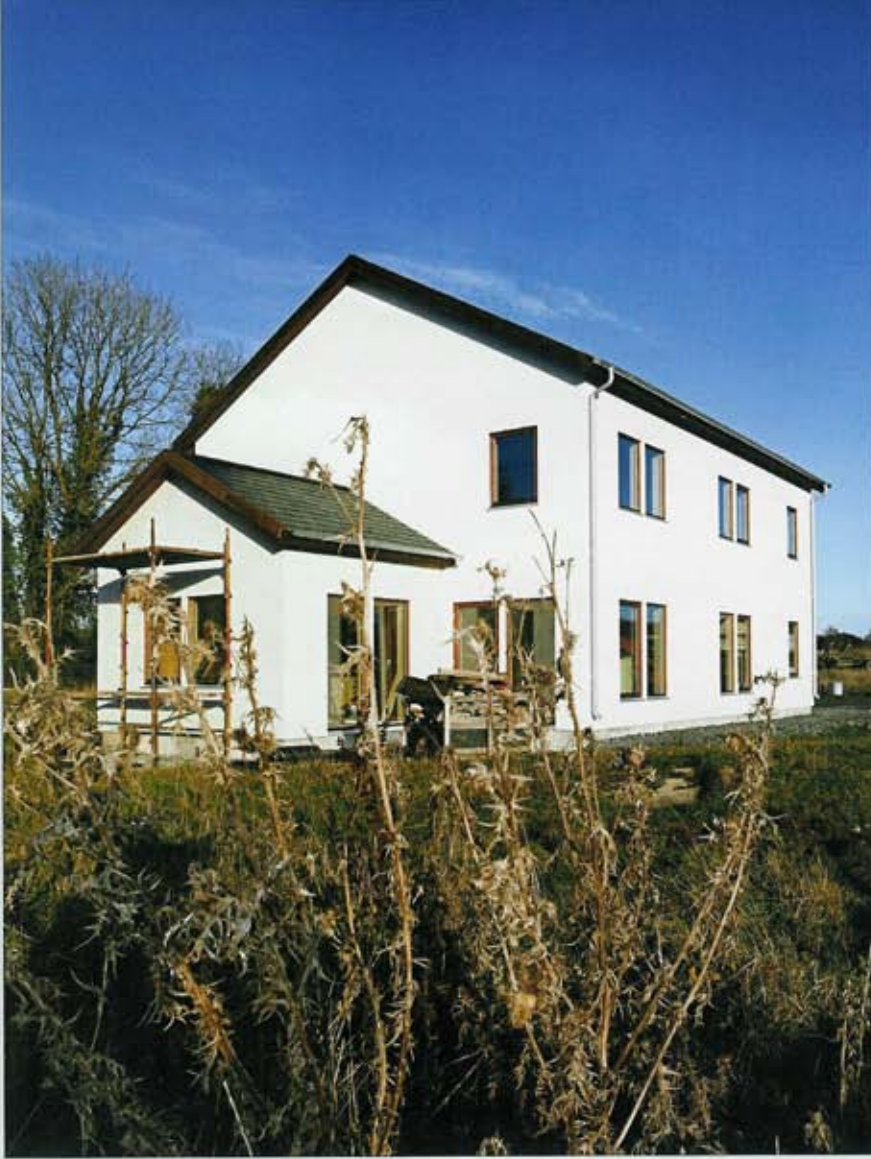
(clockwise from top left) The house's simple cube shape is designed to reduce the surface area and minimise heat loss; an automatic floor sander smooths the solid timber floors; a heat recovery unit ventilates the house; the house's timber windows are triple-glazed and argon-filled with a low-e coating
