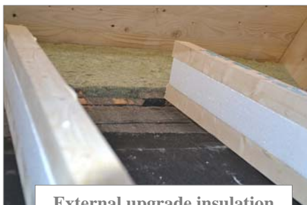
External upgrade insulation light-beams where 170mm of Rockwool is installed
